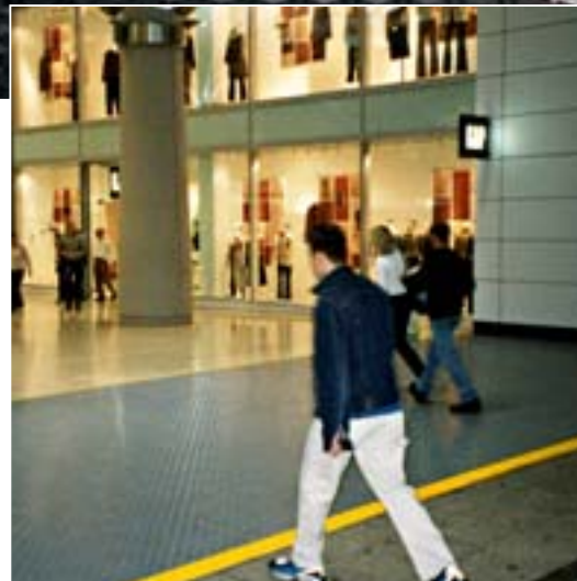
2 Shopping Centre Chequerplate is used in several areas at a large shopping centre to prevent accidents occurring as customers enter the centre from outside. The tiles effectively act as a barrier to provide an anti-slip surface and allow shoes to dry before they come into contact with the marble floor inside the shopping centre.
